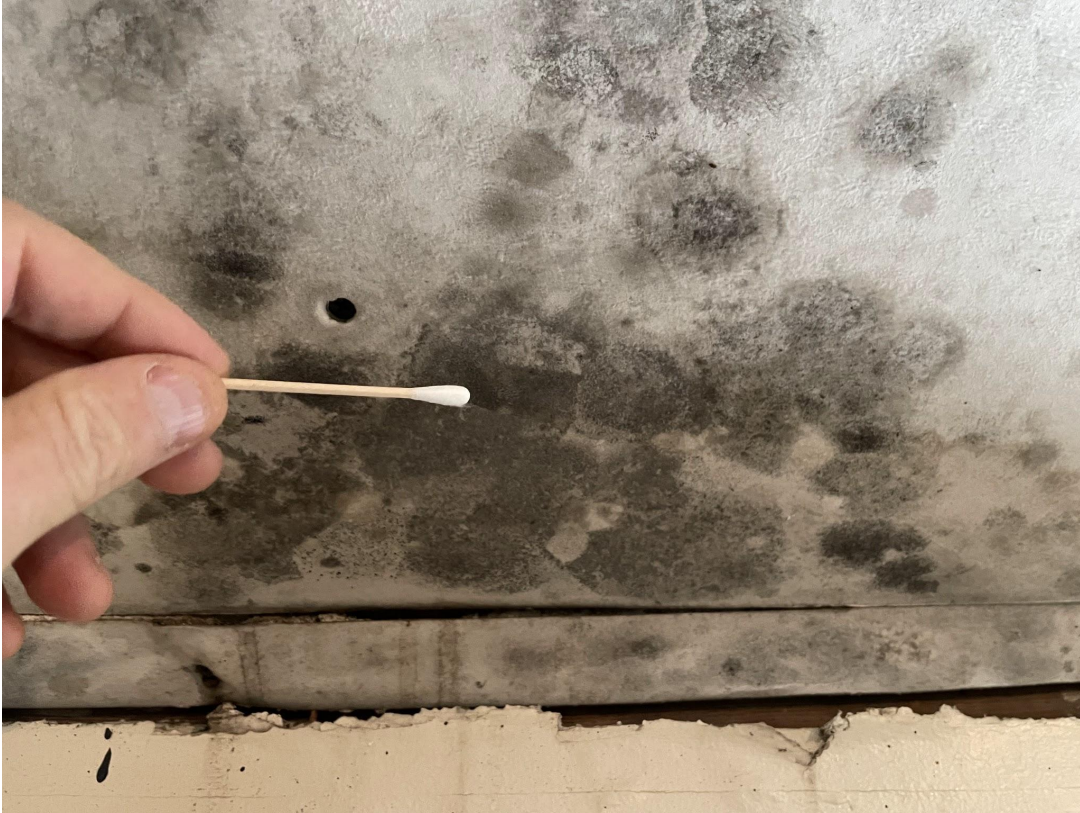
Taking a swab sample on basement drywall.
