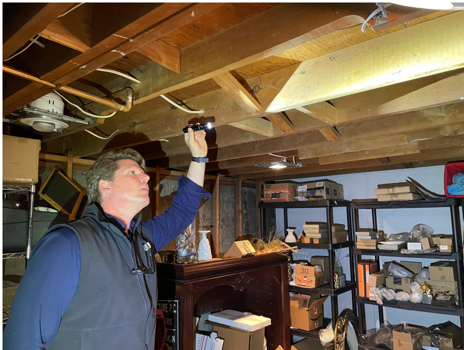
Inspecting floor structure for mold.
